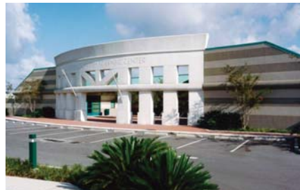
Jefferson Parish Forensic Center New Orleans, LA / 1997 Principal in Charge & Designer
